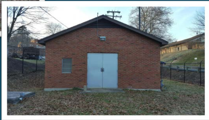
Stadium Road Pump Station - 1987
