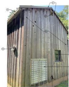
4 EXISTING CONDITIONS PHOTO BASIN SIDE OF PS3
