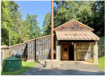
1 EXISTING CONDITIONS PHOTO FRONT OF PS3
