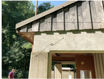
2 EXISTING CONDITIONS PHOTO BASIN SIDE OF PS3
