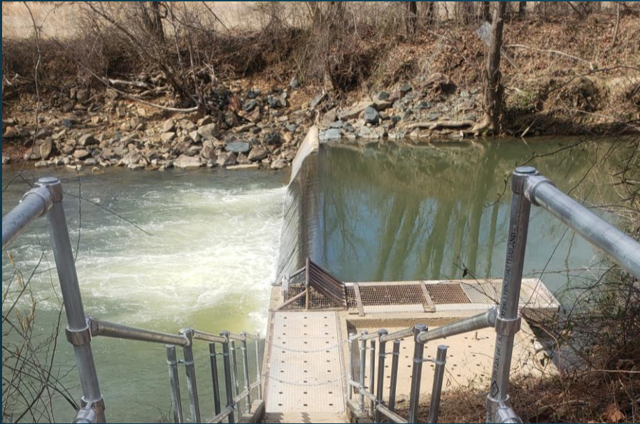
North Rivanna Low Head Dam
