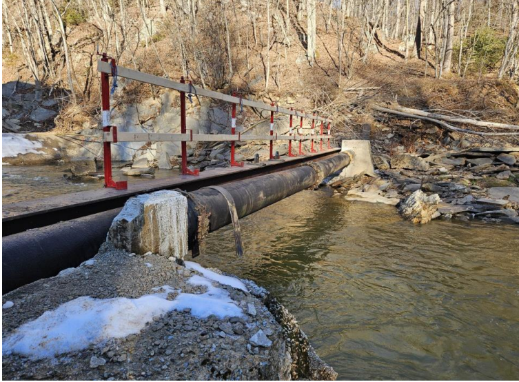
Repaired Sugar Hollow Water Line at the Mechums River Crossing.
